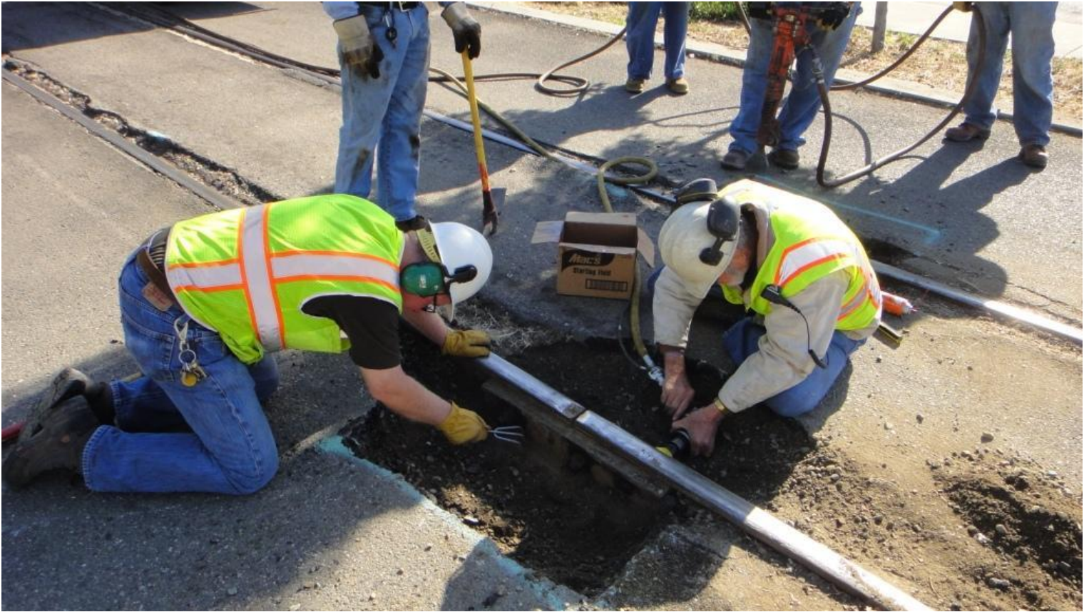
Ed clears away dirt from the west side joint-bar as Alan work with the \frac{3}{4} " impact-wrench to remove a bolt.
