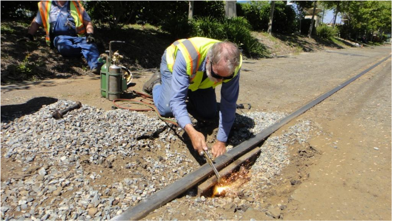
Alan torch-cuts a nut off a spinning bolt.
