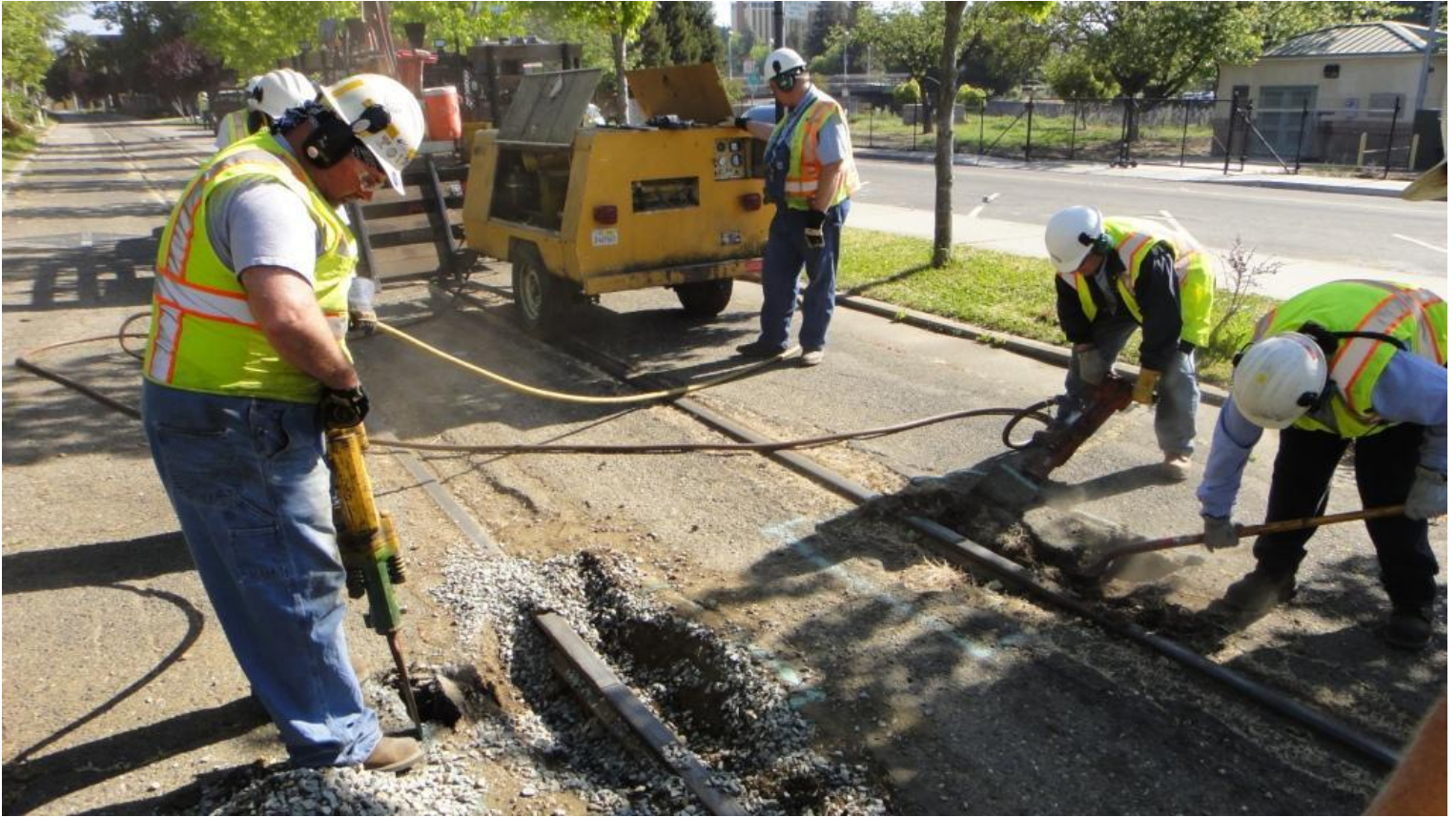
“Deliverance” MOW style: Mike F. and Mike W. in “dueling jack-hammers” while Frank shovels away the debris.
