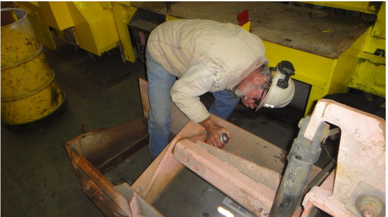
Alan applies Kroil to the bolts on the ballast regulator's wing. The plan is to expand the width of the box.
