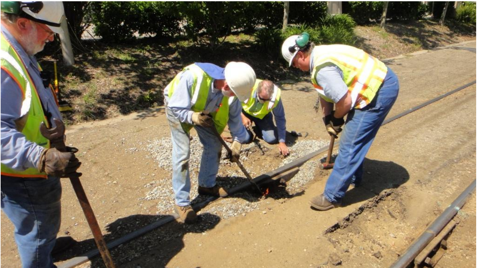
With the train having stopped-short of the red-flag at Mile Post 0.6, Mike M. and Chris strike at the cut nut with a lining bar and sledgehammer.
