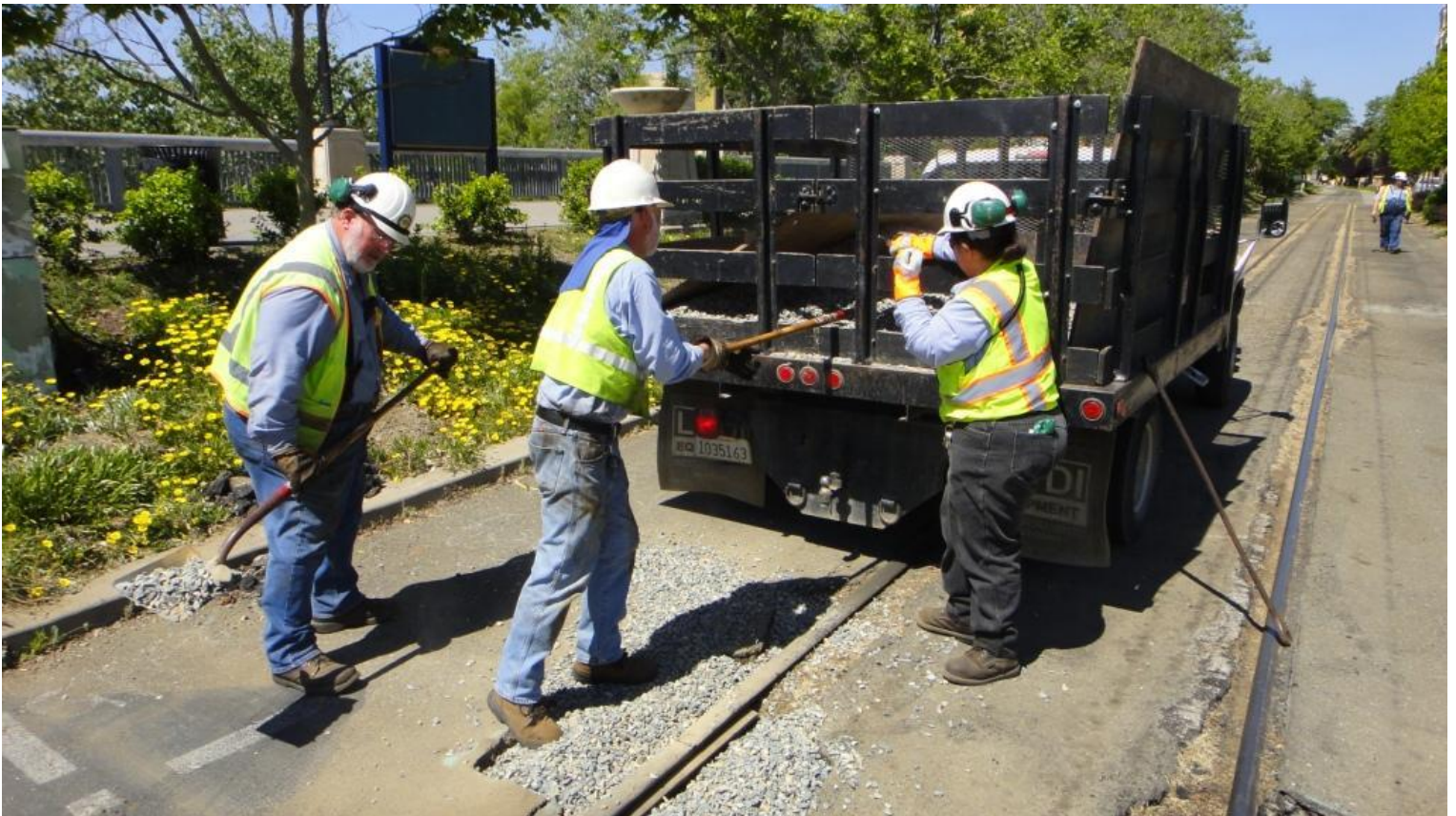
With the filling in of this joint, Frank, Mike M., and Heather complete phase-one of the Embassy Suites Alley joint servicing project.
