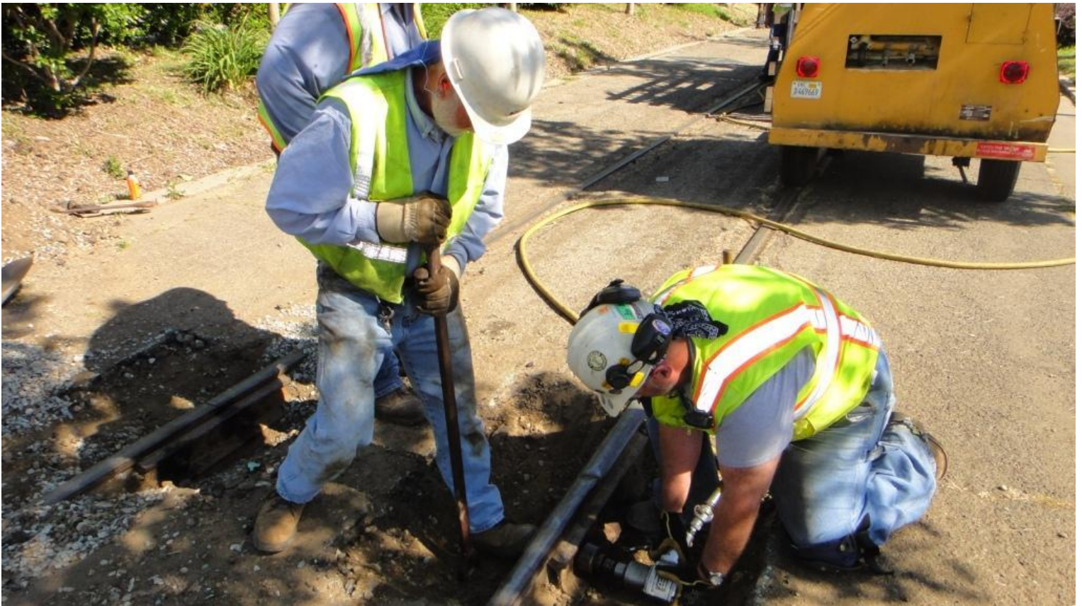
'Mike M. tries to hold in a spinning bolt as Mike F. uses the 3/4" impact on the nut.
