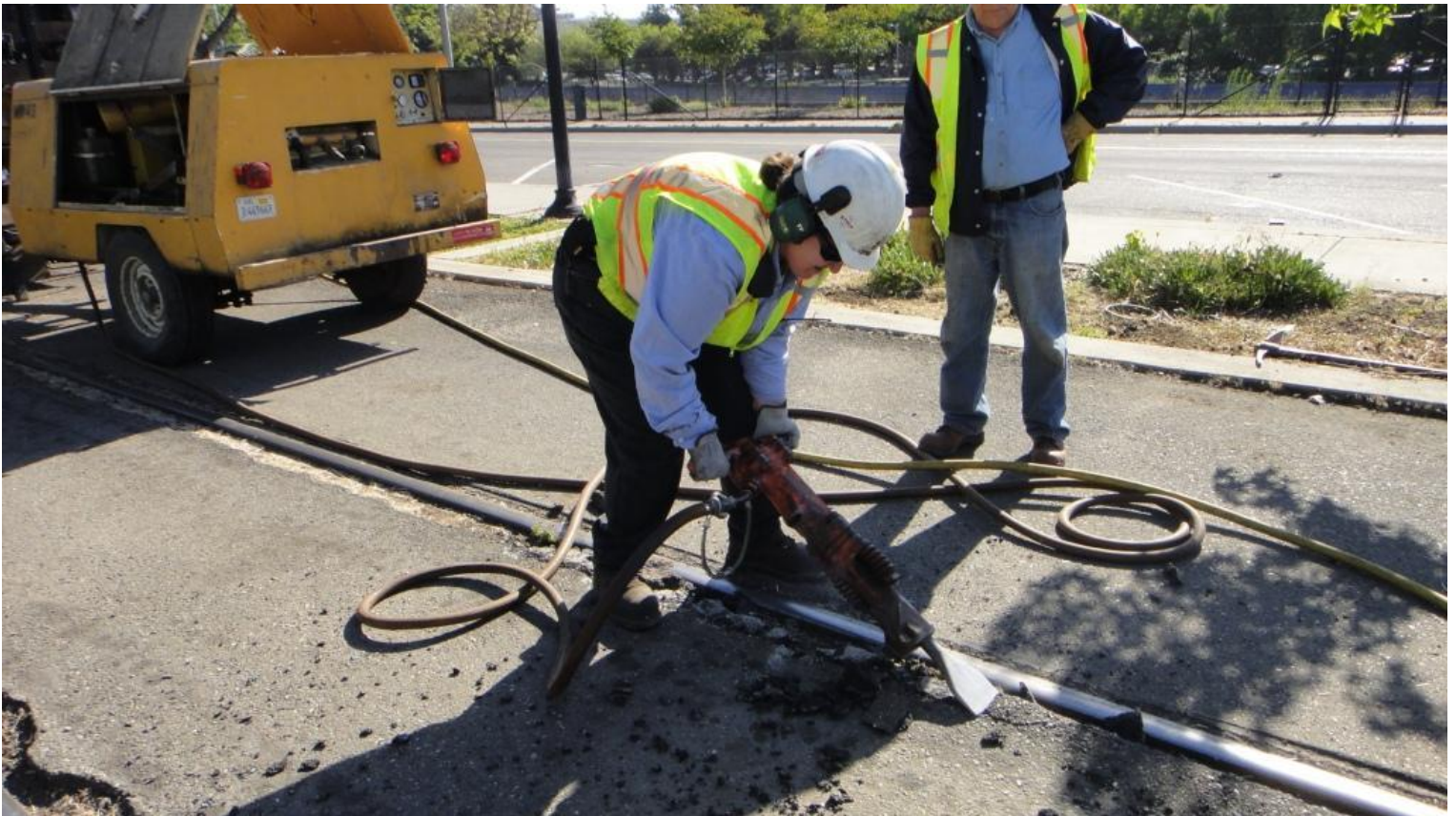
Heather jack-hammers off buckling asphalt on the gauge-side of the east rail.
