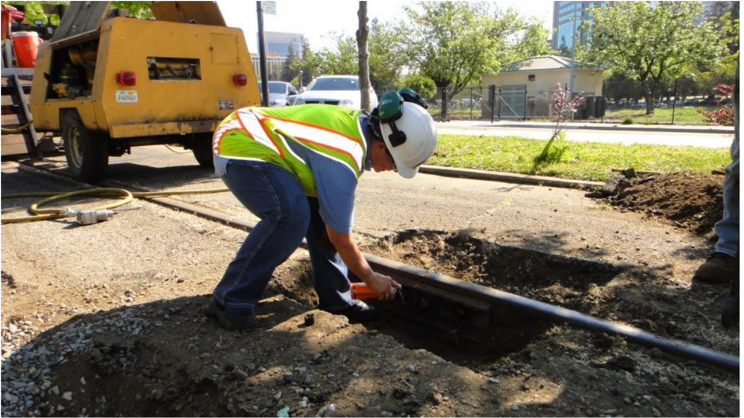
Pam sprays Kroil on the bolts.
